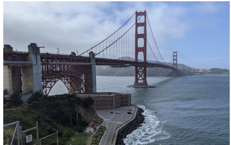
Golden Gate Bridge, California – June 2023
